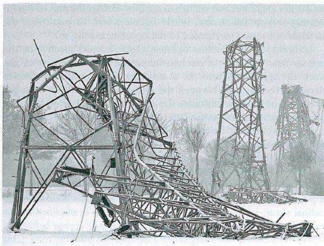
Fig. 2.3 Domino-type collapse of overhead transmission line towers triggered by ice accretion (Germany, 2005). (Source: picture-alliance/dpa/dpaweb. Photograph: Franz-Peter Tschauner, © dpa)
