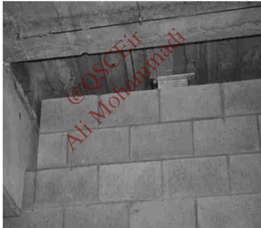
▲ 10.12 A reinforced masonry infill wall separated from surrounding structure. Note the horizontal and vertical gap (to beam) and a galvanized steel bracket resisting out-of-plane forces yet allowing in-plane movement. Office building, Wellington.
