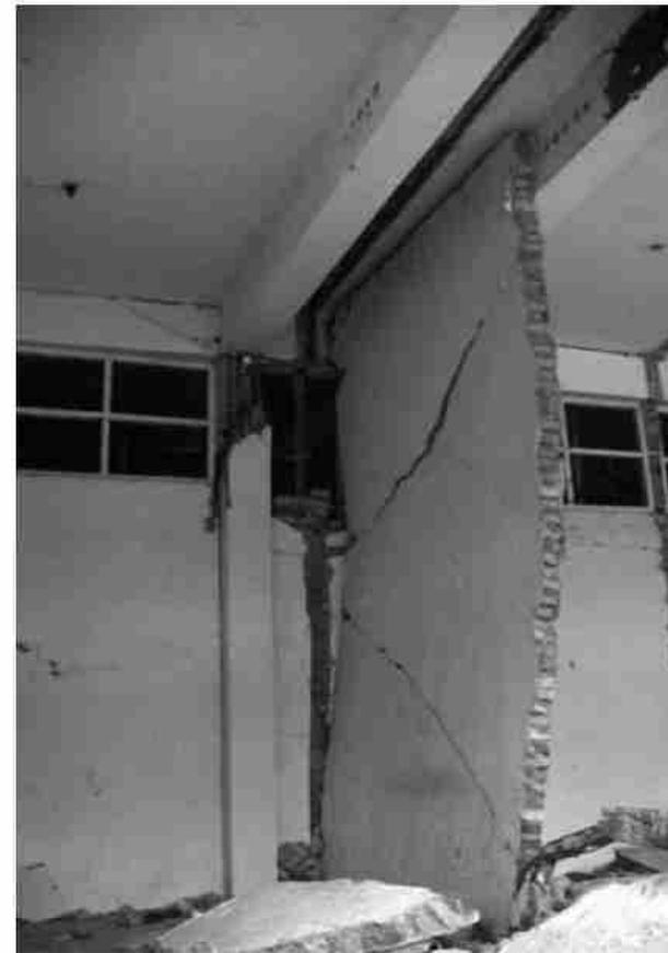
▲ 10.13 Partial out-of-plane collapse of an unreinforced masonry infill wall. Commercial building, Tarutung, Indonesia, 1987 Sumatra earthquake.
