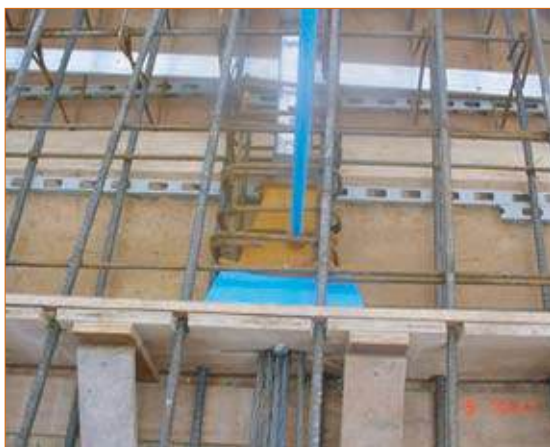
Figure 7.38 Bursting reinforcement for a typical live end in a post-tensioned slab (courtesy of Sir Robert McAlpine Ltd)
