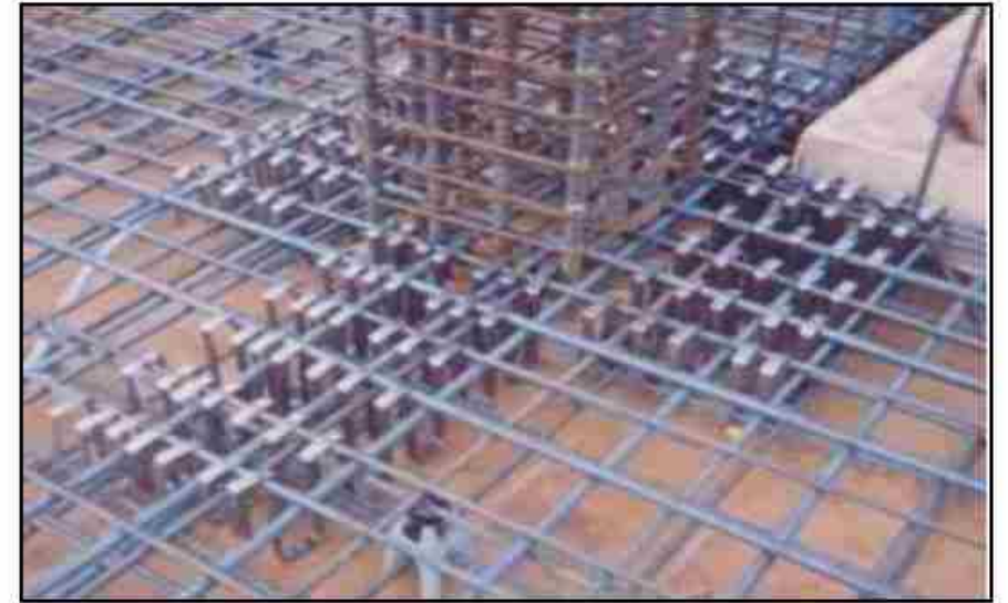
Fig. 2.14: (a) Shear Band, and (b) Placement around column
