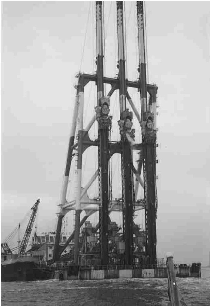
Figure 16.36 Construction of sand compaction pile in Yokohama, Japan Harbor (Courtesy of E. C. Shin, University of Incheon, Korea)
