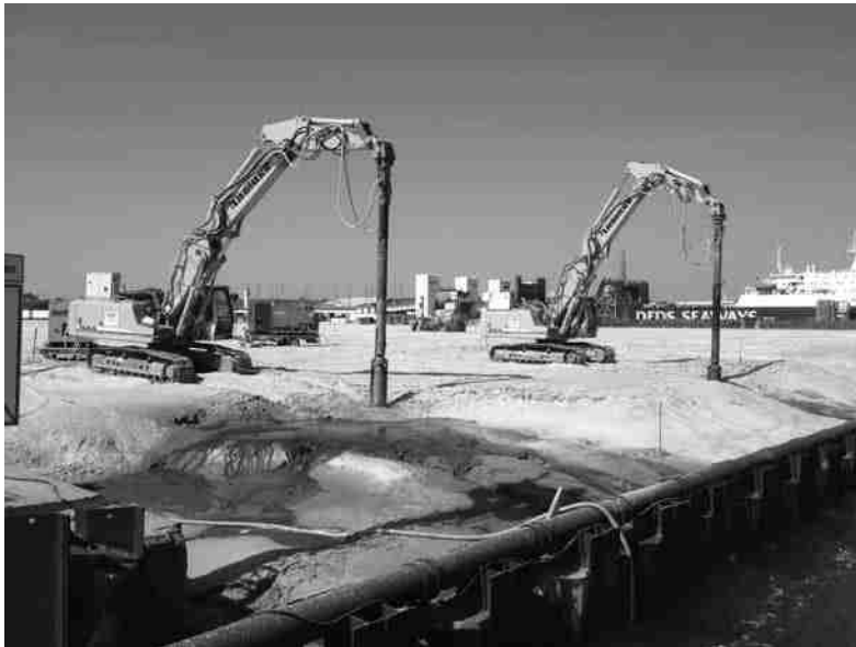
Figure 16.32 Construction of a stone column [DGI-Menard (USA).]
