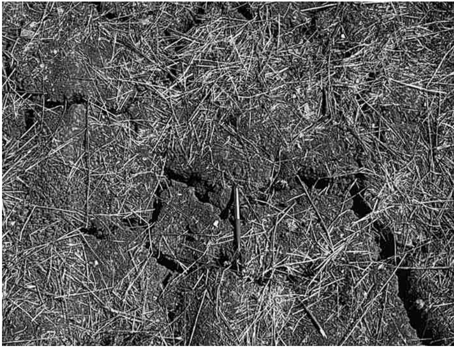
Figure 11.9 Shrinkage cracks on ground surface in a clay weathered from Eagle Ford shale formation in the Dallas-Fort Worth area (Courtesy of Thomas M. Petry, Missouri University of Science and Technology, Rolla, Missouri)
