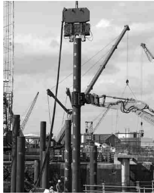
Figure 9.7 (continued) Pile-driving equipment: (e) vibratory pile driver; (f) photograph of a vibratory pile driver (Courtesy of Reinforced Earth Company, Reston, Virginia)
