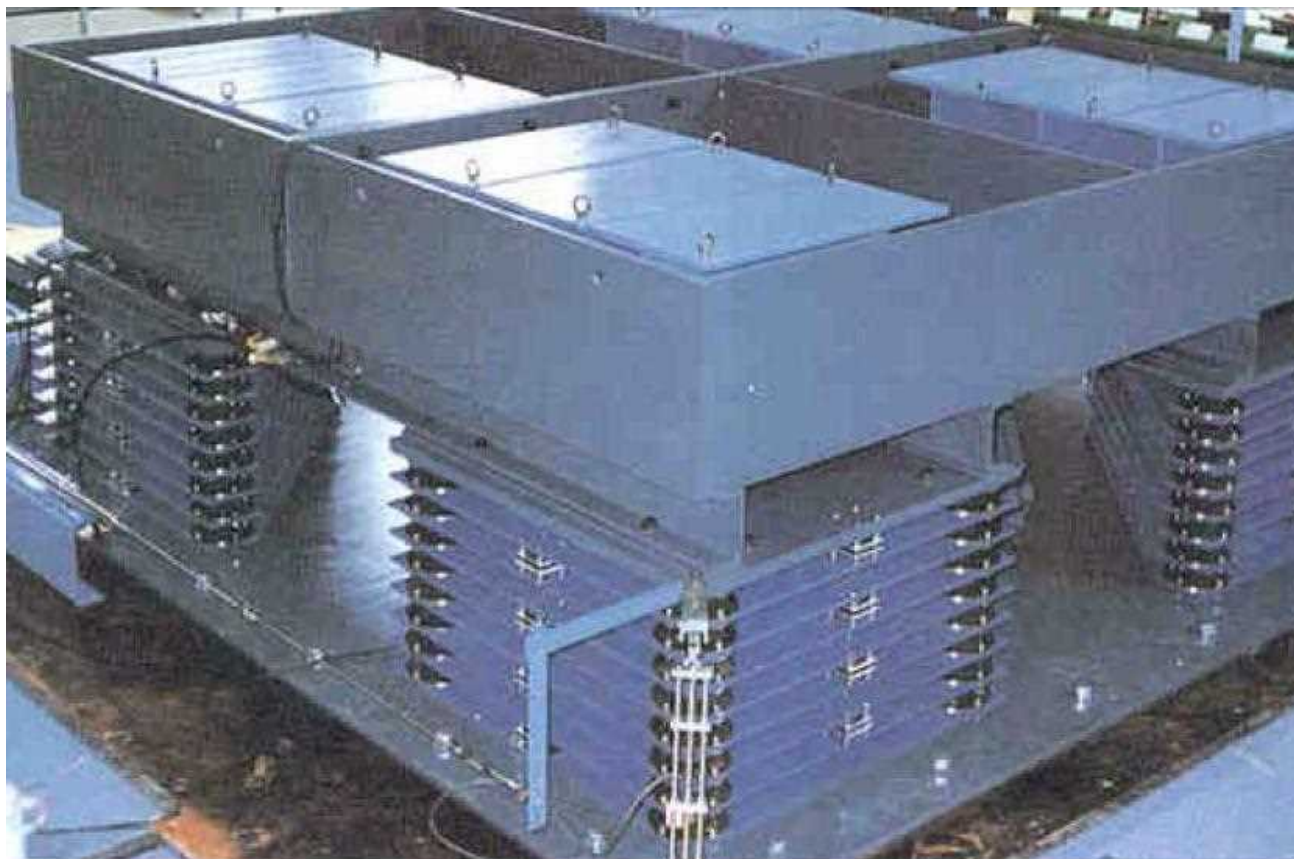
Fig. 4.6: Tuned mass damper - Huis Ten Bosch Tower, Nagasaki.
