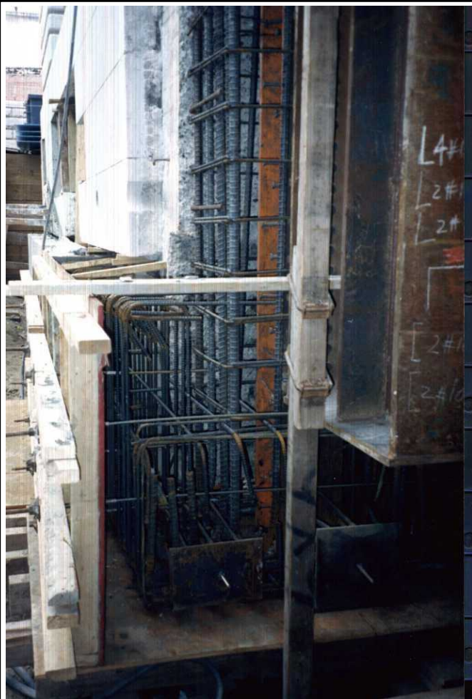
Cutting hole for jacks and column removal
