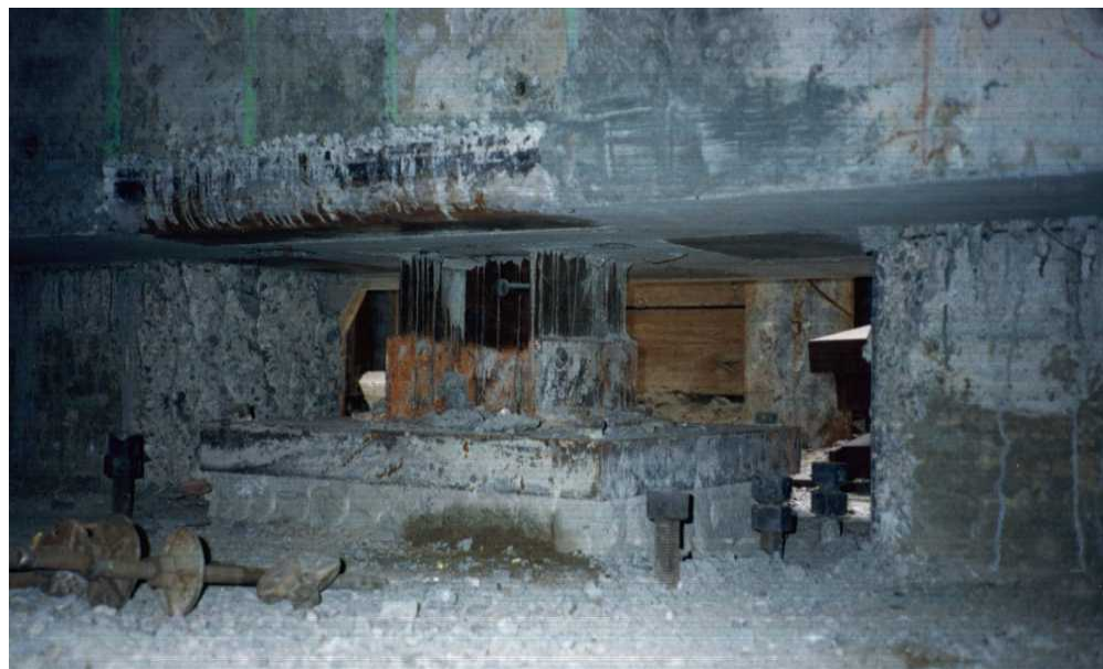
Cutting hole for jacks and column removal
