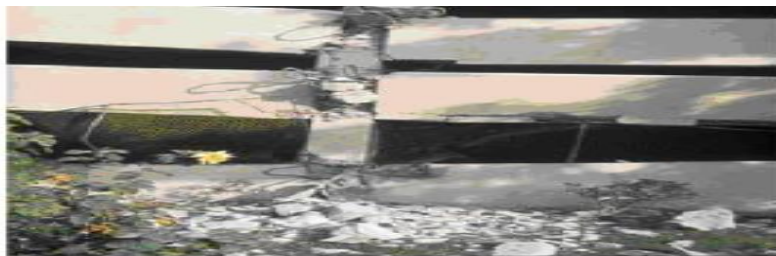
Column failures
